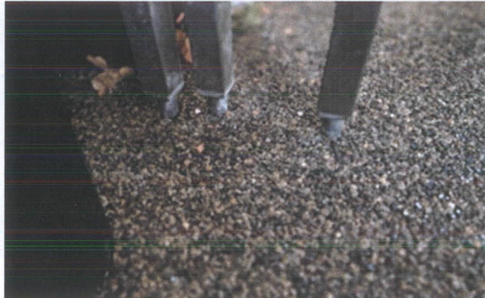
Figure 10 showing bar feet on ground
