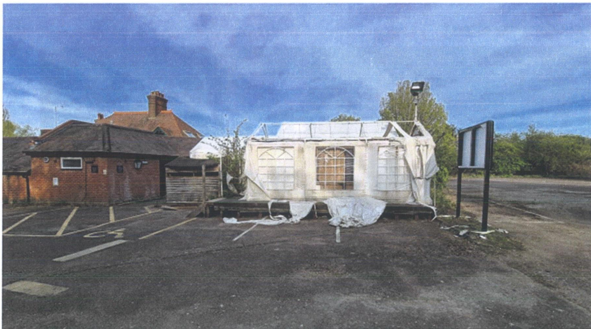
Figure 14 (showing the former timber structure which we replaced under planning approval)
